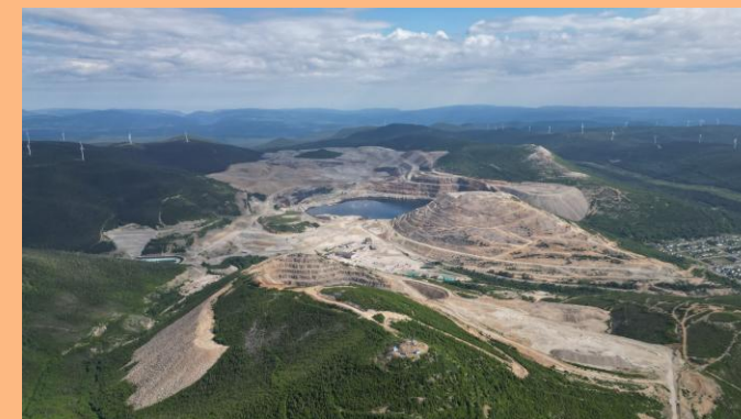
ONE OF CANADA'S LARGEST COPPER PROJECTS
