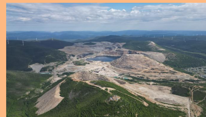
ONE OF CANADA'S LARGEST COPPER PROJECTS
