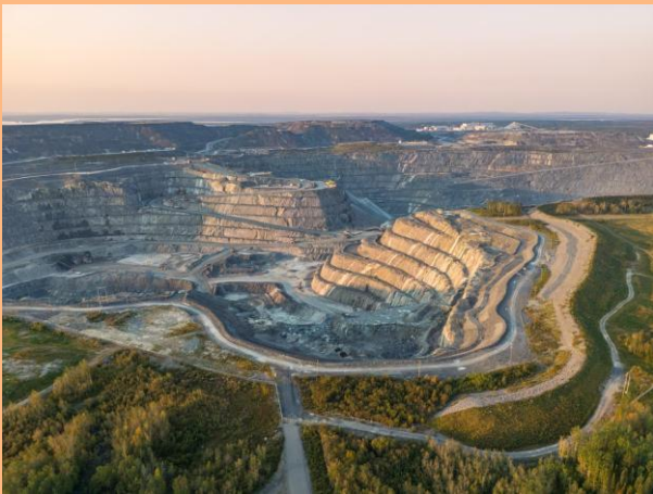
CANADA'S LARGEST GOLD MINE
