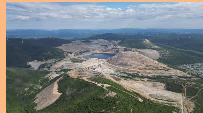
ONE OF CANADA'S LARGEST COPPER PROJECTS
