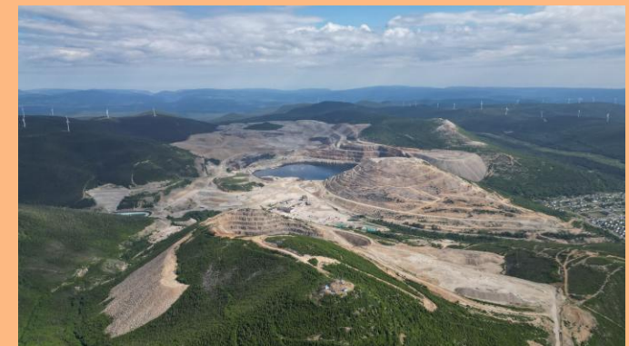
ONE OF CANADA'S LARGEST COPPER PROJECTS
