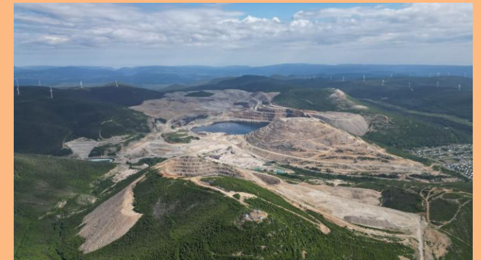
ONE OF CANADA'S LARGEST COPPER PROJECTS
